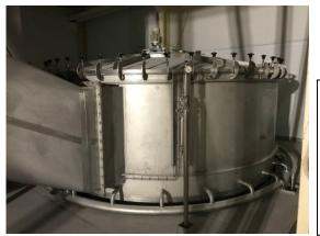
The new bag filter uses 10-meter bags, the existing had only 7-meter bags, but the diameter of the new bag filter is almost the same, so it was no problem fitting it in."
